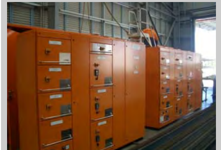
Consep's automation systems
